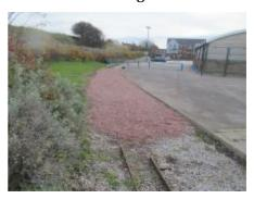
Over the winter many hours have been spent improving RMR's **track**. On the section shown above flooding caused the ballast to become contaminated with sand. We lifted the track here and Welsh Water then dug out the stone and replaced it with fresh ballast, following which the track was reinstated.
