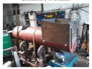
The boiler for RMR *Joan* continues to make steady progress. In the photograph the new outer firebox plates are being lined up with the existing boiler barrel. Parts of the RMR **Cagney** locomotive have also departed to the Midlands for mechanical attention.
