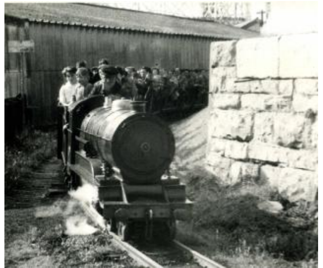
This undated photo shows a train on the original (pre 1969) railway weaving its way around the corner of the old sea wall. The wall is still there now, but of course the building and the big dipper (both in the background) are only memories. The train would have been six cars and seems to be full – as per usual in that period.
